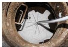
Razorooter II is the only diquat-based herbicide registered by the U.S. Environmental Protection Agency for controlling nuisance tree roots in sanitary sewer systems, and received a classification of "evidence of non-carcinogenicity for humans."
