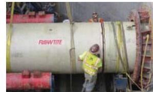
Many challenges face the water and wastewater pipeline industry for open cut, slip-rehab, or trenchless jacking installations. The globally proven product, Flowtite FRP pipe, can often be the answer with non-corrosive gravity and pressure class pipe (462-psi max), various stiffness, various joint lengths (50 foot maximum), lightweight, quality solutions.
