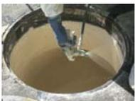
Sauereisen SewerGard® No. 210X is a protective lining specifically formulated for municipal wastewater environments. SewerGard® No. 210X provides a chemical-
