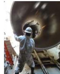
HOBAS pipe is suitable for virtually every installation method of new construction and rehab. The centrifugally cast, fiberglass-rein-
