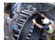
DuroMaxx® SRPE pipe provides a proven trenchless installation method for
