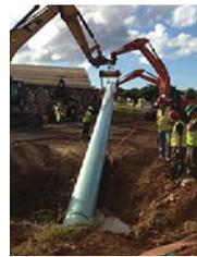
monolithic, fully-restrained, gasket-free, leak-free piping system ideal for trenchless or conventional "open-cut" installations.
