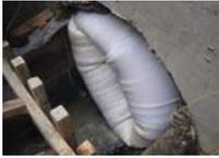
designed for use with reinforcement containing tubes for CIPP pressure liners. Short term burst strength results of these liners have approached 1,300 psi. These resins are corrosion resistant, have high tensile strength properties, are as easy to process as standard CIPP liners and come in a styrene containing or styrene free versions.
