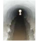
Shotcrete offers an alternative to the 'digging and replacing' of damaged culverts, sewers, and storm drains. Shotcrete provides all the benefits and structural properties of traditional concrete, less expensive, and environmentally friendly. This trenchless repair, using Shotcrete, eliminates road closures, disruption of traffic, and expensive 'above ground' bypassing pumping.
